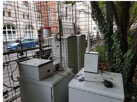
Fig. 10: The prototype unit placed on the right equipment container in the garden of Marienschule towards the roadside of Bundesstrasse B14
