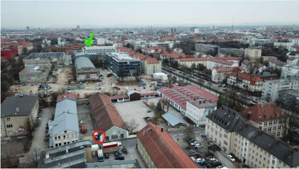
Figure 61: Position of the Twin-SDS measurement box at Maker Lab Munich (red circle) with respect to the LfU reference station in Munich Lothstrasse (green arrow)
