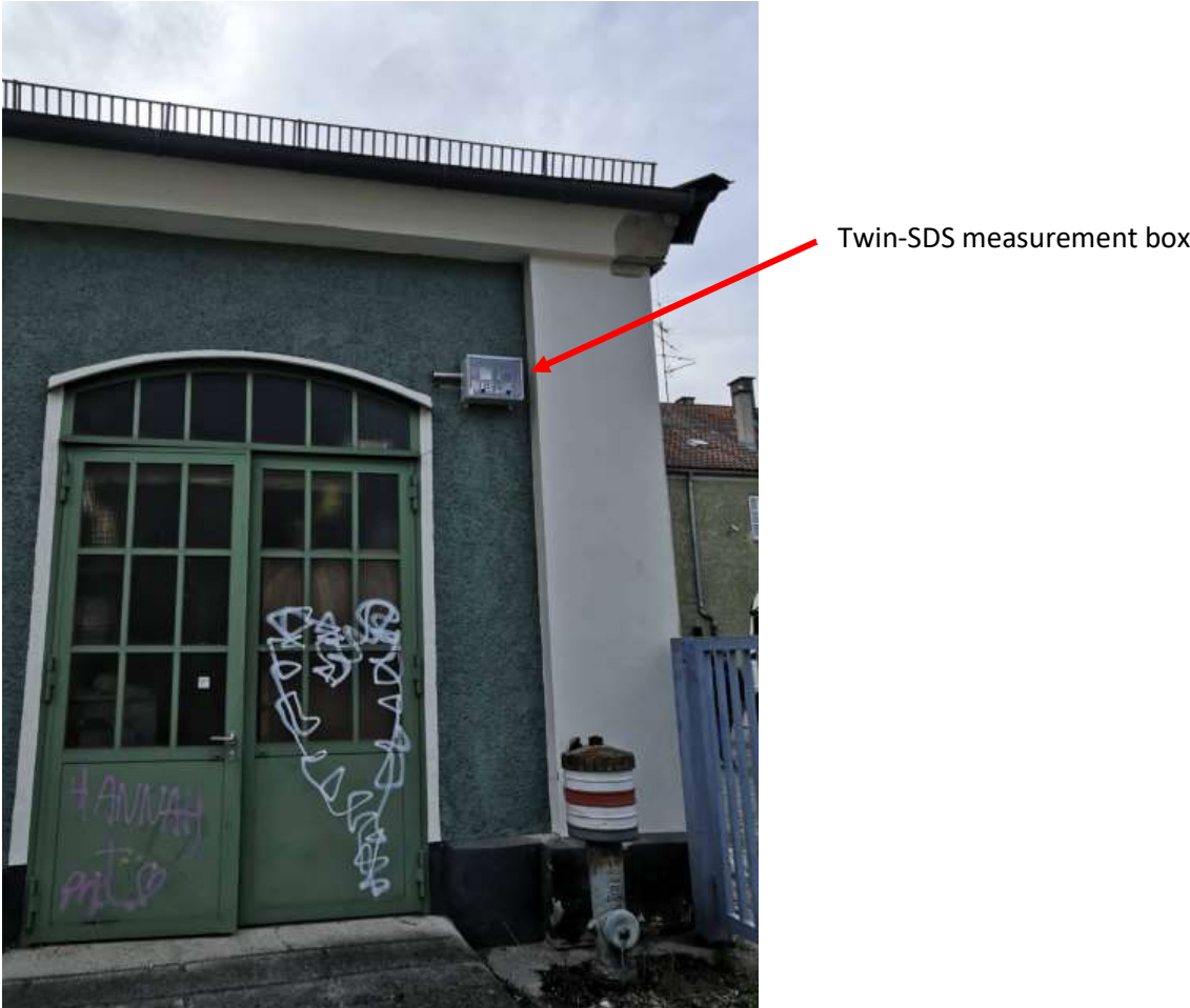
Figure 62: Position of the Twin-SDS measurement box used for the co-location measurement at the wall of a building opposite to Munich Maker Lab e.V.
